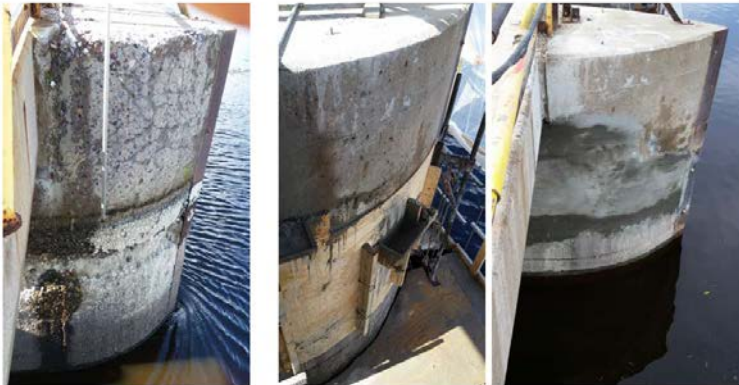
The three stages of repair of the concrete piers.
